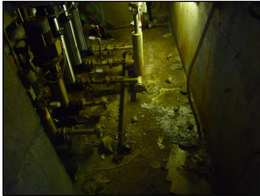
Plate 68 Brewhouse subterranean plant room
