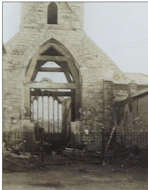
Plate 35 Northern elevation of Tower 1928
