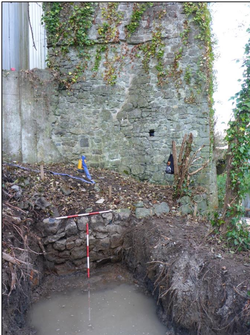
Plate 31 Revetment wall at Evan's Tower
