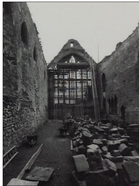
Plate 36 Work in progress to East Window
