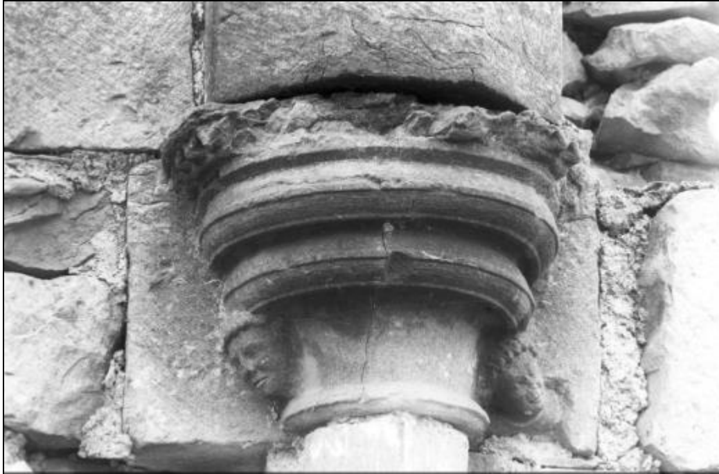
Plate 10, The Stalley Collection , Bell capital with dogtooth on (damaged) abacus and head carvings to left and right of shaft, www.gothicpast.com
