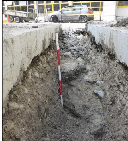
Plate 29 Monitoring ESB trench, culvert section 1
